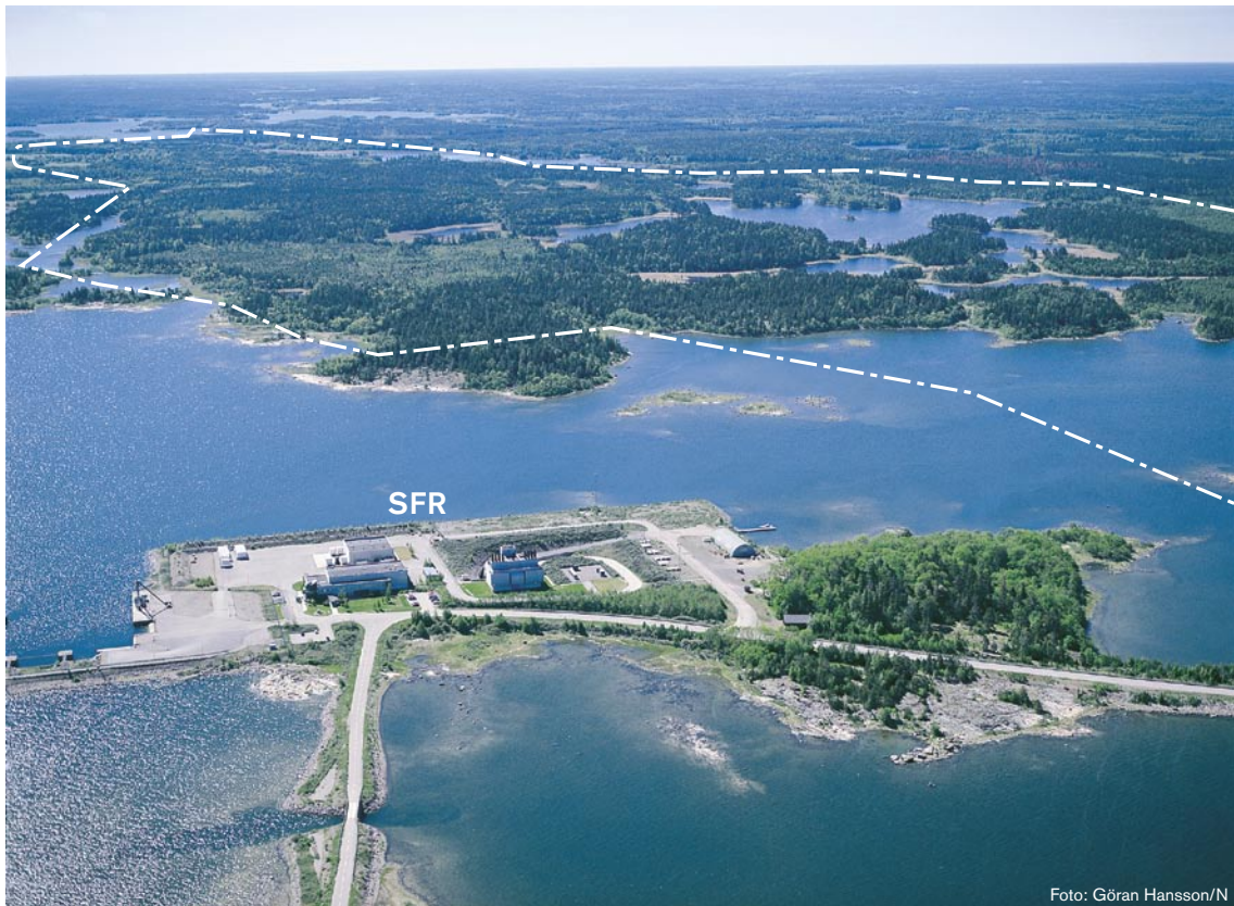
Figure 1-5. General view towards the south of the Forsmark site showing the outline (dotted line) of a portion of the investigated area. The surface infrastructure associated with Forsmark SFR Facility is in the foreground.
