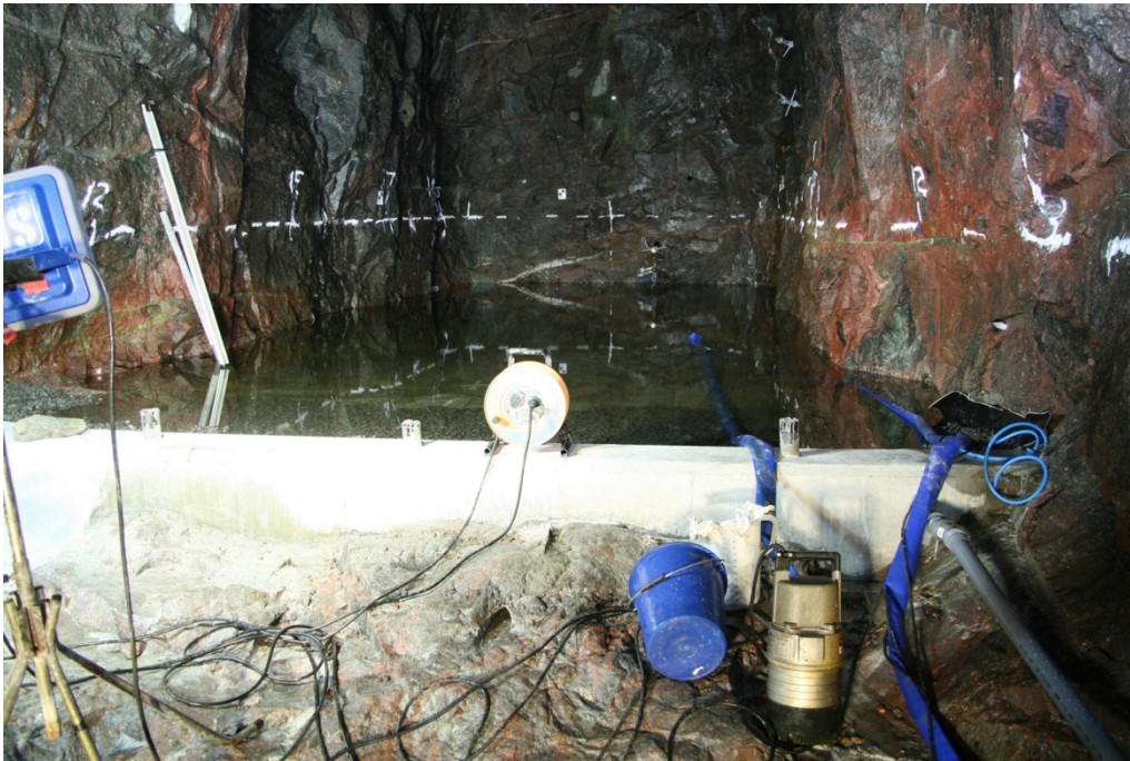
Figure 4-1. Water filled measuring weir in the project Sealing of Tunnel at Great Depth.
