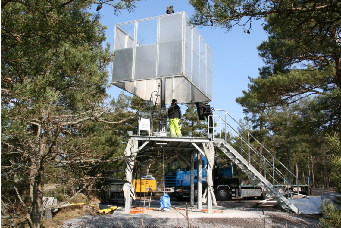
Figure 2-2. Mobilising for retrieval of monitoring equipment from borehole KAS09.
