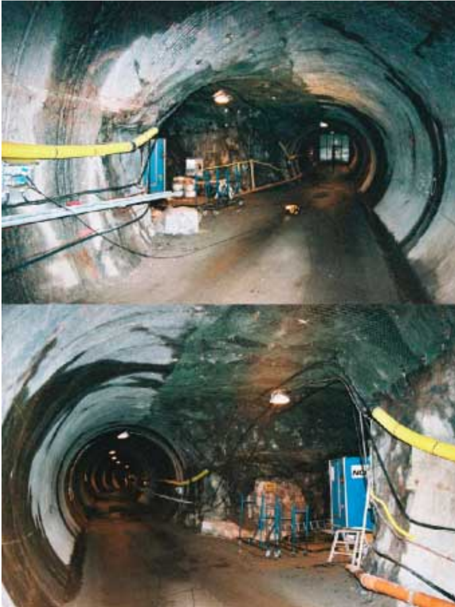
Figure 4-15. Top photograph taken looking east and bottom photograph taken looking west shows the entrance of niche 3419B. Note the intact TBM-tunnel on both sides of the niche.
