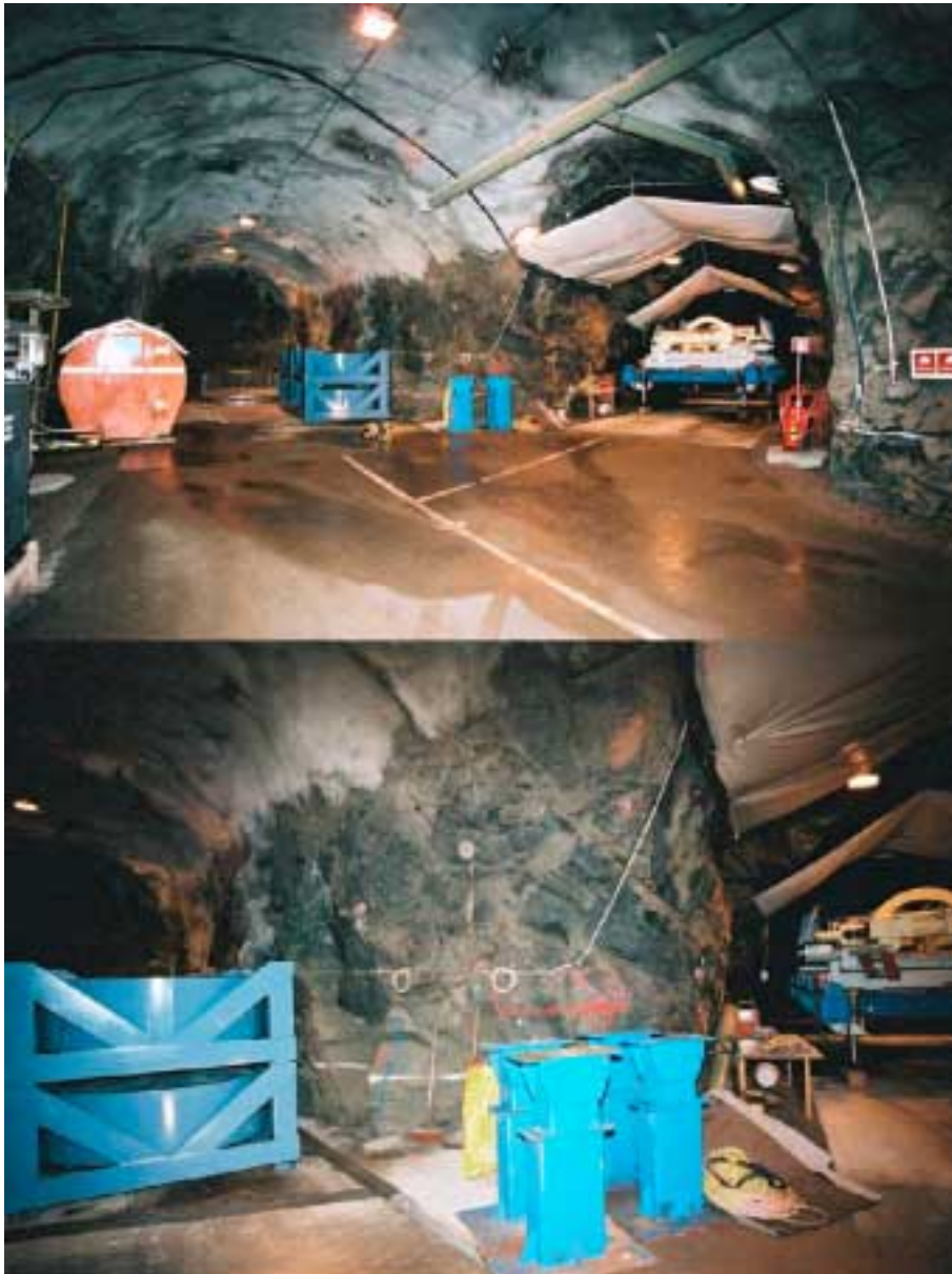
Figure 4-10. Photograph of the T ASD-tunnel to the left and T ASO-tunnel to the right. Bottom picture is a close-up on the pillar between the tunnels. The pillar is rather unaffected by its low confinement and is sparsely bolted.
