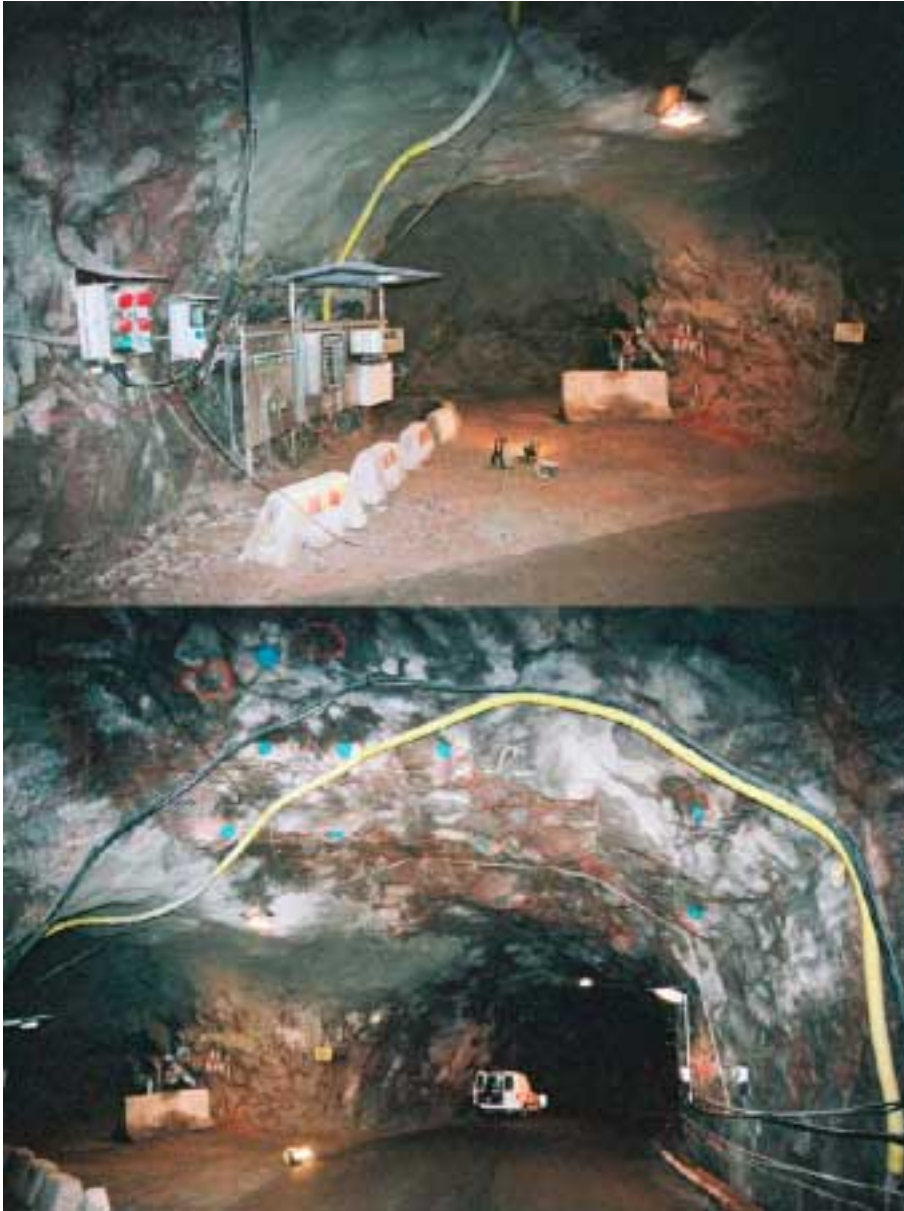
Figure 4-6. Top photograph shows the entrance to NASA 3009A indicating the dull corners. Bottom photograph is taken down the main tunnel with the niche to the left. The blue discs are washers to the rock bolts.
