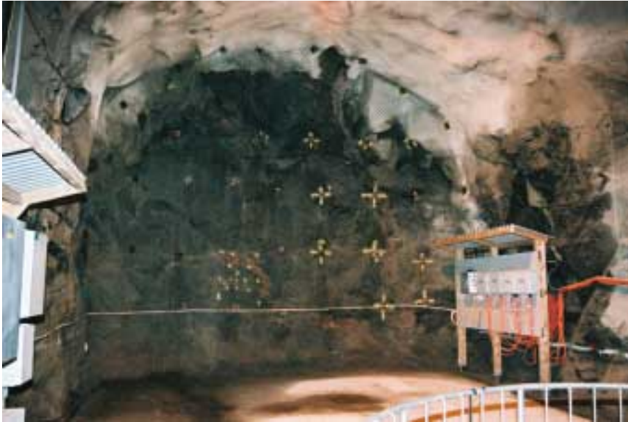
Figure 4-11. Photograph of the front of the D-tunnel and its support.
