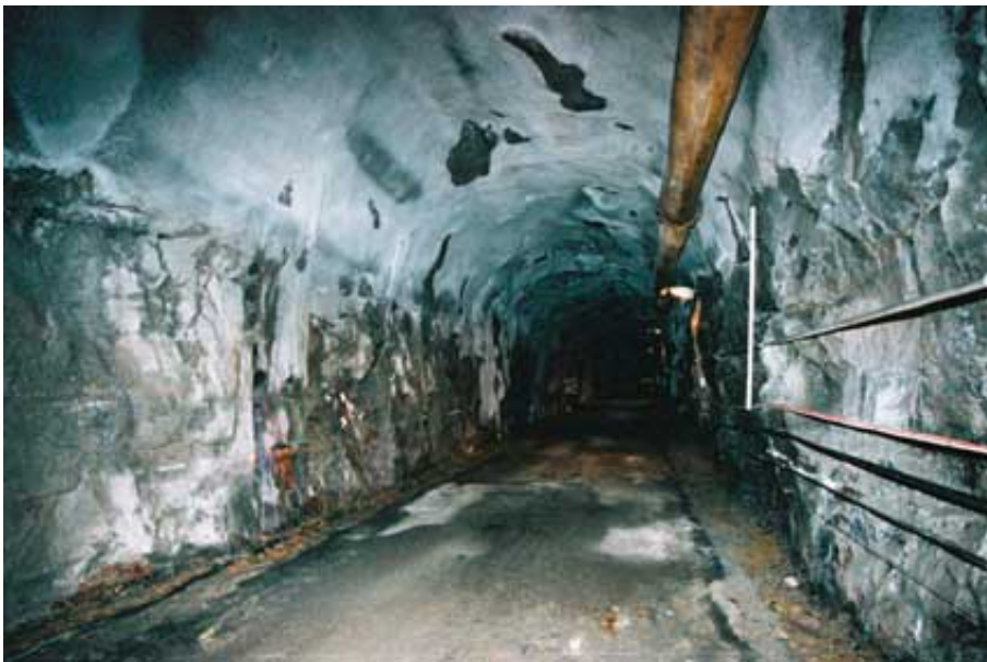
Figure 4-28. Top photograph is taken down the TASF-tunnel.
