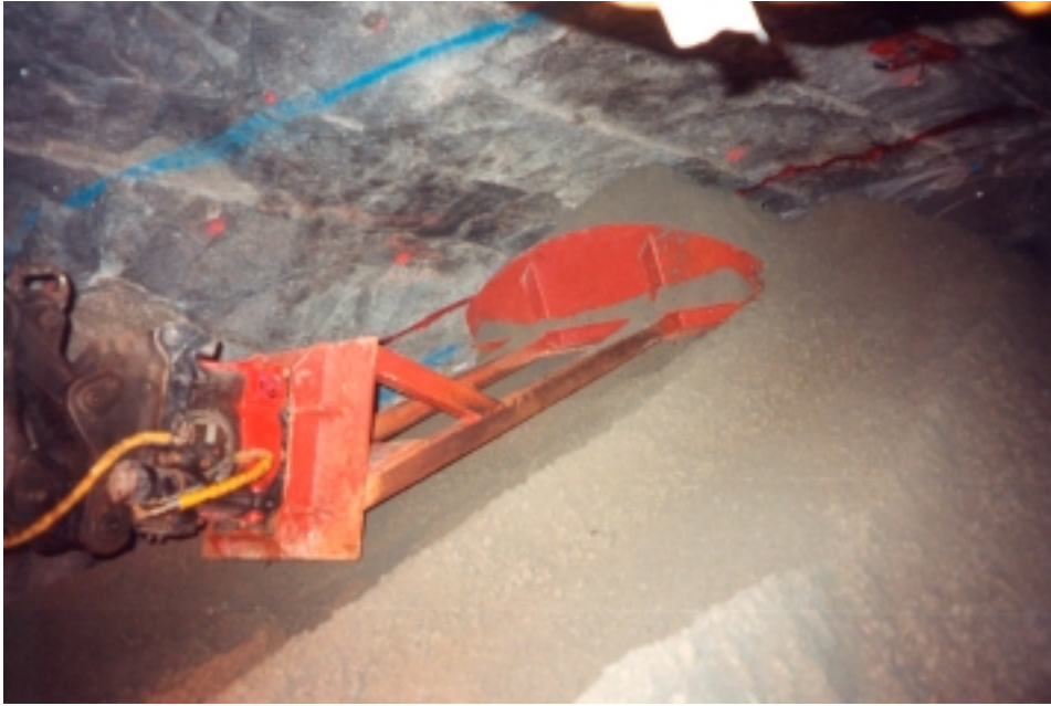
Figure 7-11. Pushing the material in place.
