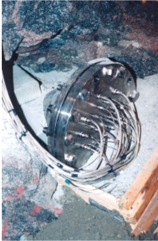
Figure 7-6. Exit of an installed cable package in the test tunnel.
