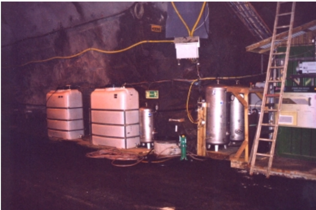
Figure 11-30. Photo of pressure vessels and storage tanks.
