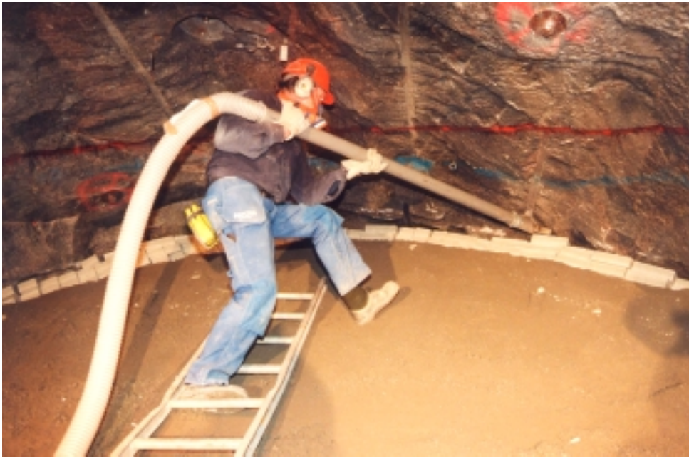
Figure 7-14. Emplacement of pellets
