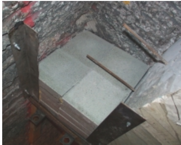
Figure 12-11. Left: Positions for test emplacement. Right: Blocks in position V3. The reinforcement bars sticking out of the concrete rim were intended as support for the blocks, but were never used. Prior to the real emplacement they were removed.
