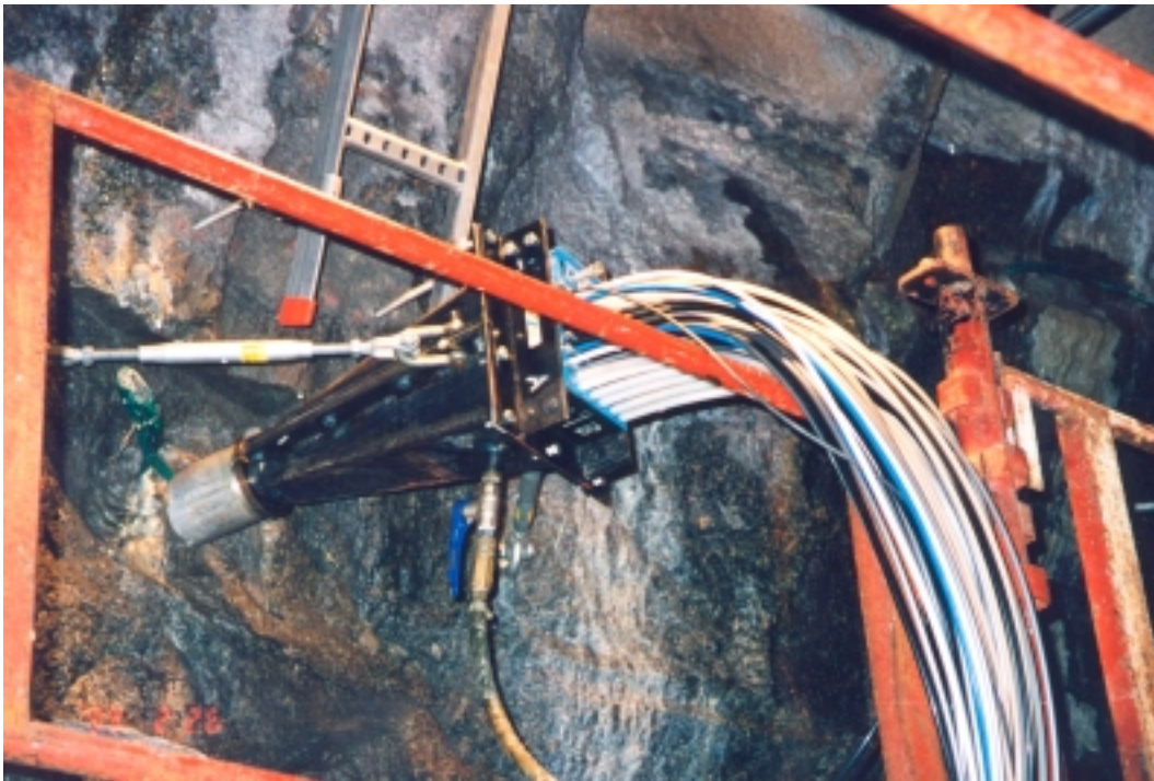
Figure 9-10. Temporary seal for the third leakage test series
