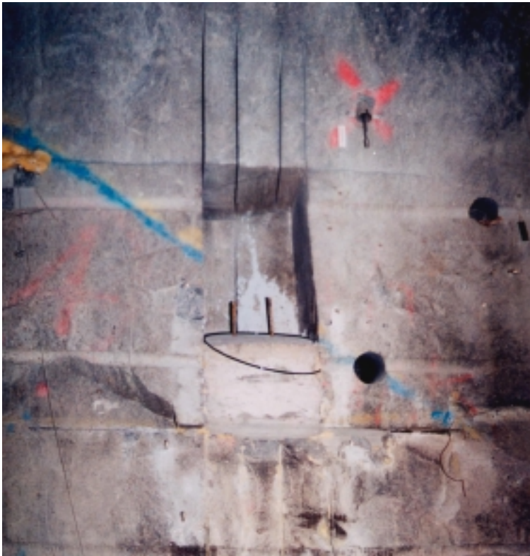
Figure 5-6. Sealing of a slot
