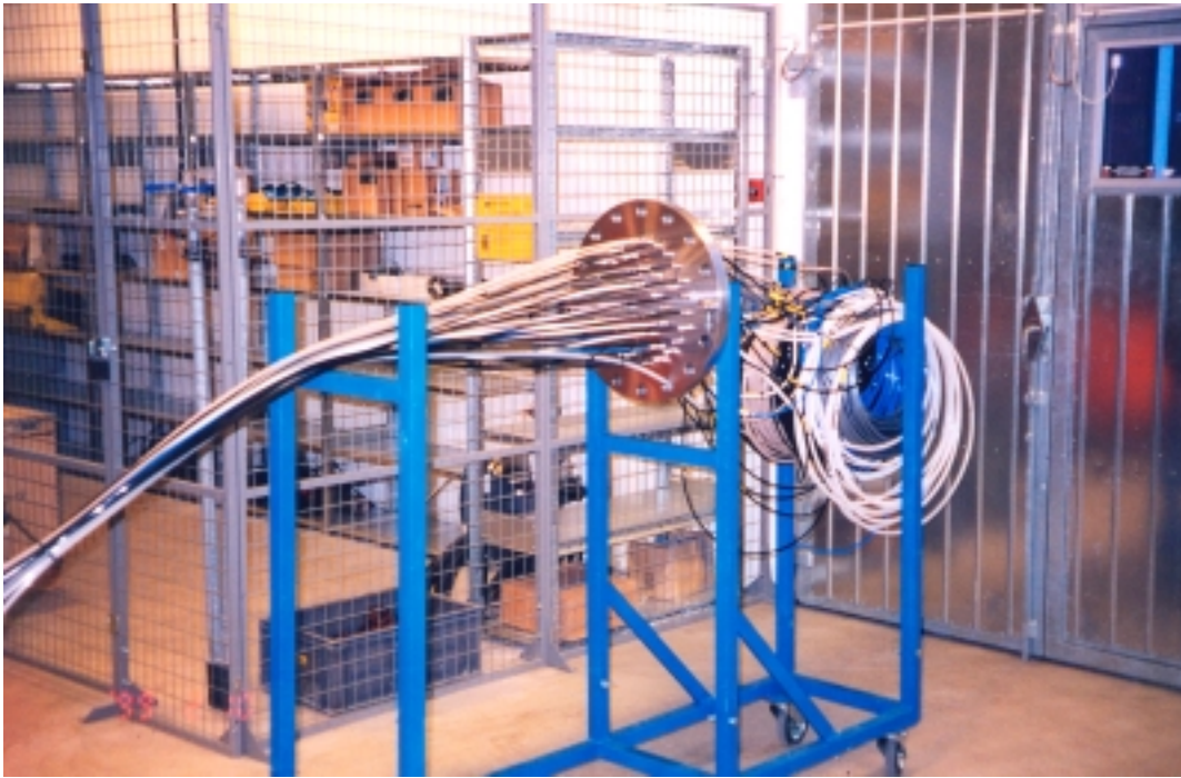
Figure 9-6. The rack with an assembly of cables and a flange.
