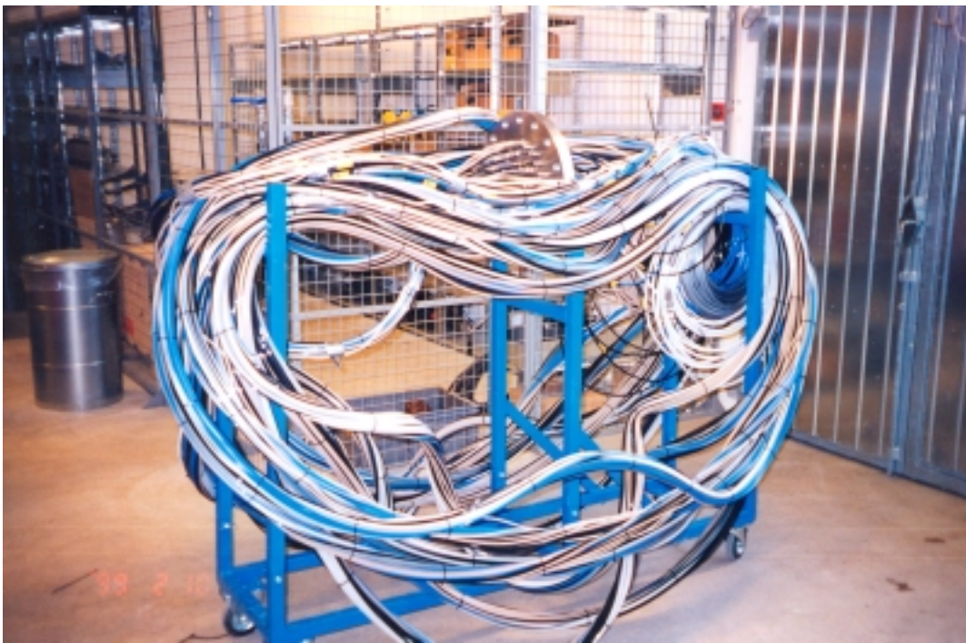
Figure 9-7. A cable bundle on the rack ready for installation.
