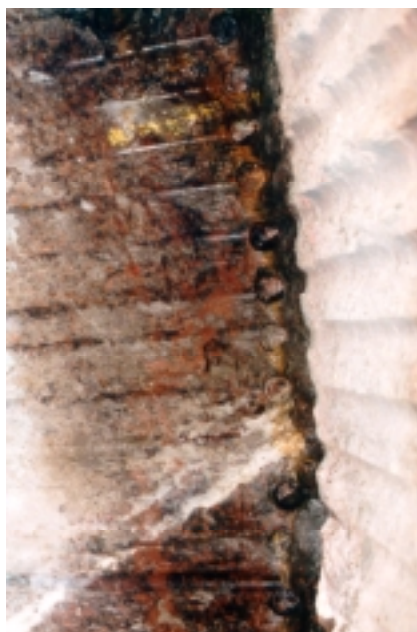
Figure 12-7. Slot surfaces after reworking.
