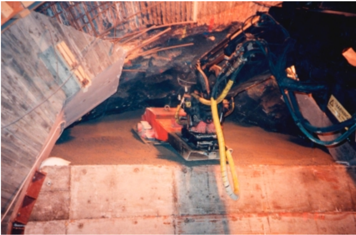
Figure 7-19. Backfilling against the concrete beams
