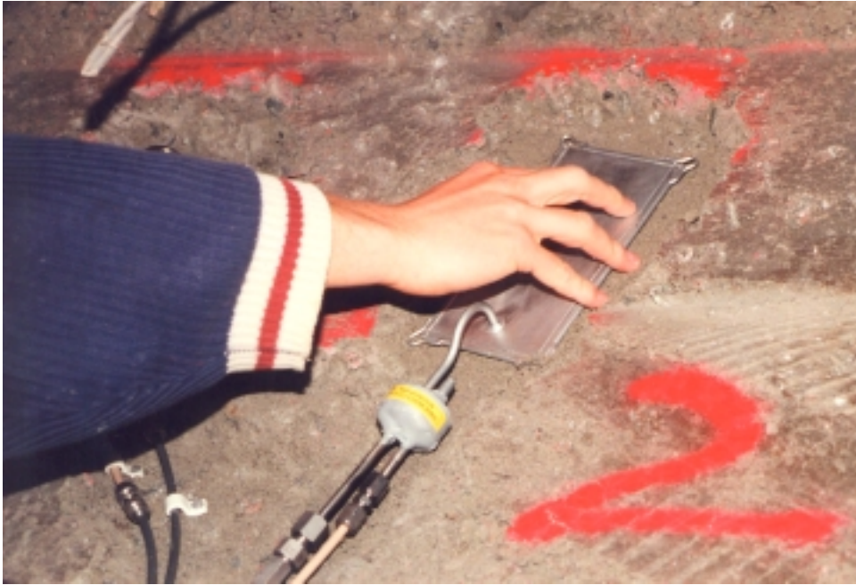
Figure 11-6. Installation of a Glötzl total pressure cell in the backfill.
