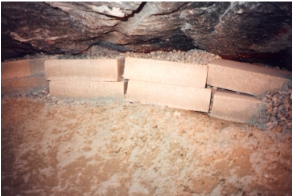
Figure 7-15. Blocks and pellets placed in the slot at the roof.
