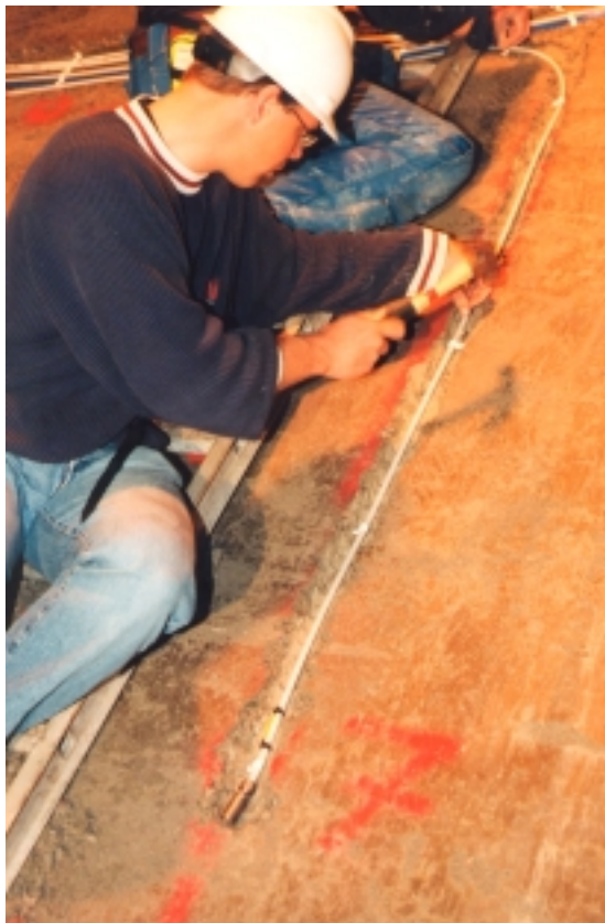
Figure 7-7. Installation of cables on the surface of a backfill layer
