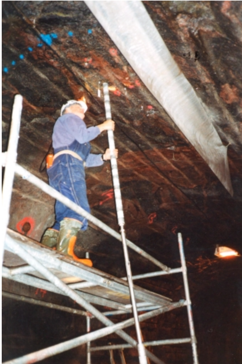
Figure 5-2. Installation of bentonite packers
