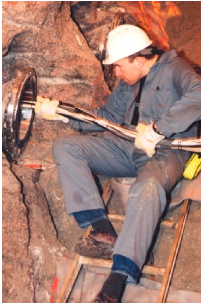
Figure 9-8. Guidance of a cable package through a cone and tube.
