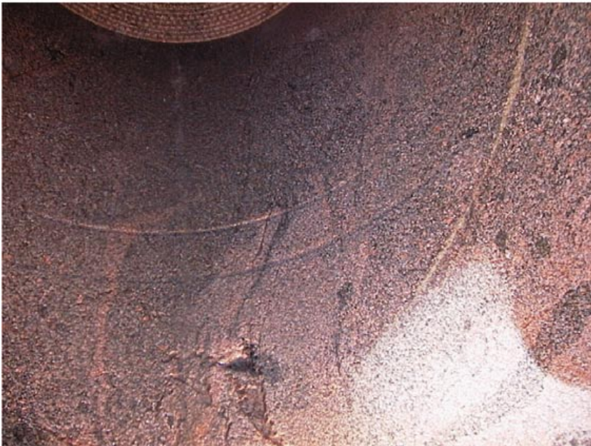
Figure 3-7. Some typical types of surface unevenness in deposition drift: cavities on the drift roof (top) and rims shaped grooves and a notch (above). Photos by J. Autio.
