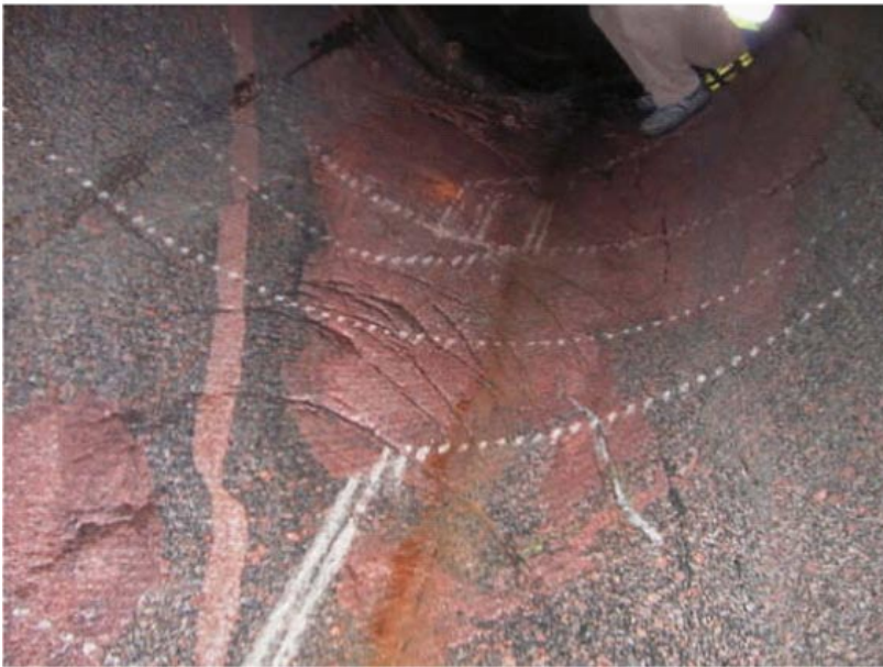
Figure 3-6. Some typical types of surface unevenness in deposition drift: rifle type grooves on the drift wall (top) and notches at fracture intersections on the floor (above).
