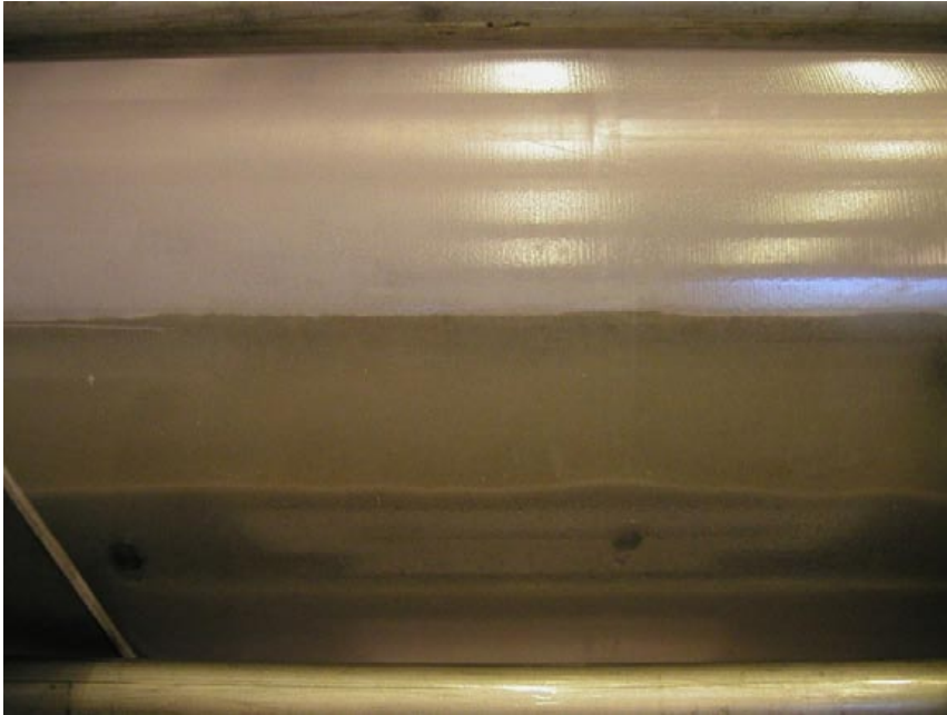
Figure 3-31. Picture taken during the pre-wetting of the outer slot. Water is filled halfway up and bentonite has loosened from the blocks and settled down in the bottom.
