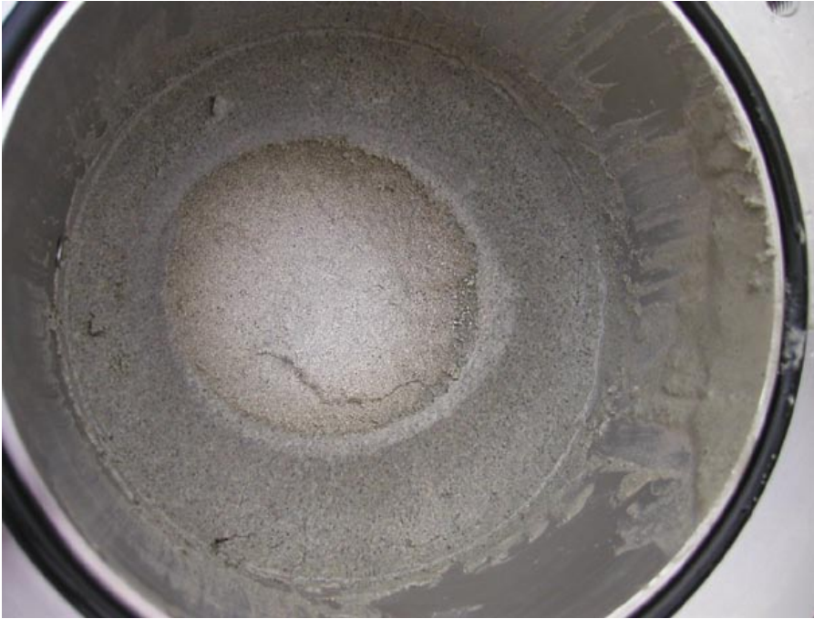
Figure 3-15. Picture showing the surface just inside the supercontainer dummy. The ring shaped “active surface” can be well distinguished.
