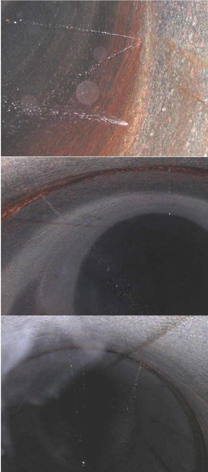
Figure 4-11. Example of spraying inflow points in the KBS-3H demonstration drift at Äspö. Photo by J Autio.
