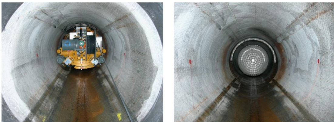
Figure 8-15. The deposition machine has entered the deposition drift (left). The supercontainer is placed approximately 20 m into the deposition drift (right.)
