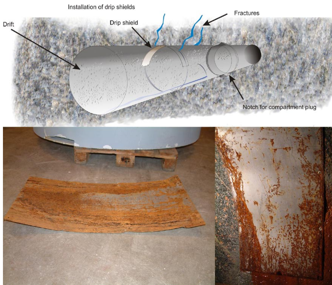
Figure 4-12. Principle of using drip shields (top) and as attached to the demonstration drift at Äspö (above right) and after detachment on the floor (above left). Photos by H. Wimelius.
