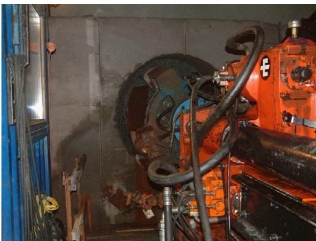
Figure 4-44. The start of reaming the pilot hole to full diameter.
