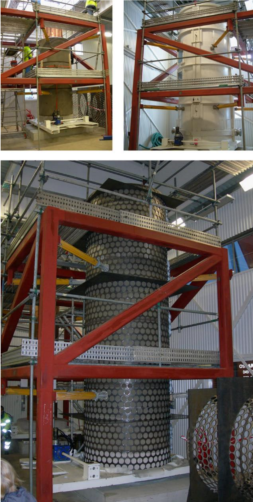
Figure 4-32. Supercontainer assembly at Äspö.
