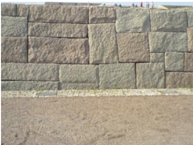
Figure 2-10. Masonry of granite blocks.
