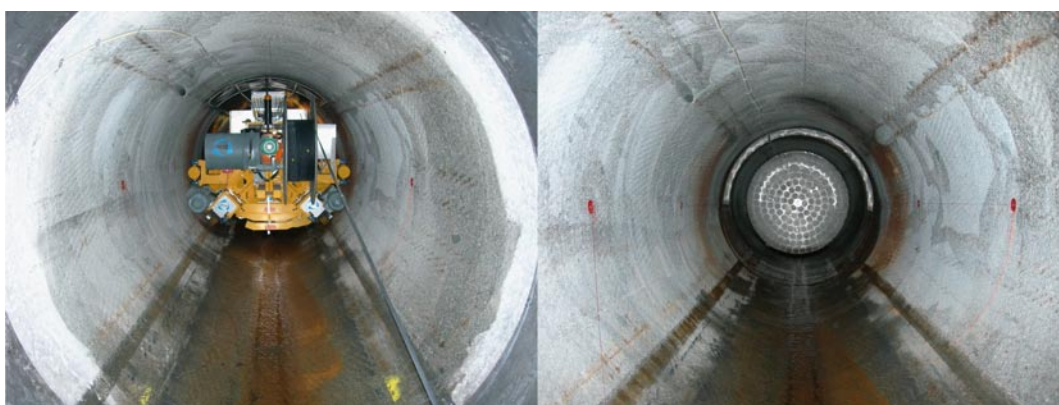
Figure 6-8. The deposition machine has entered the deposition drift (left). The supercontainer is placed approximately 20 m into the deposition drift (right).
