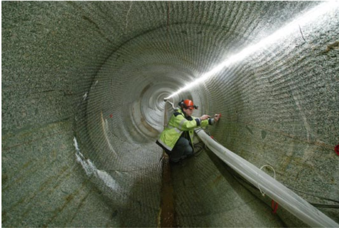
Figure 4-16. Photo taken inside the drift at Äspö HRL showing the good rock conditions and the surface roughness in the drift wall.
