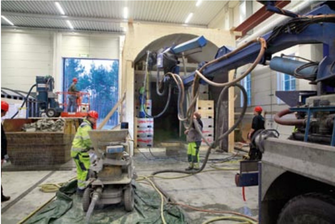
Figure 4-8. Pellet filling by using shotcreting technique.
