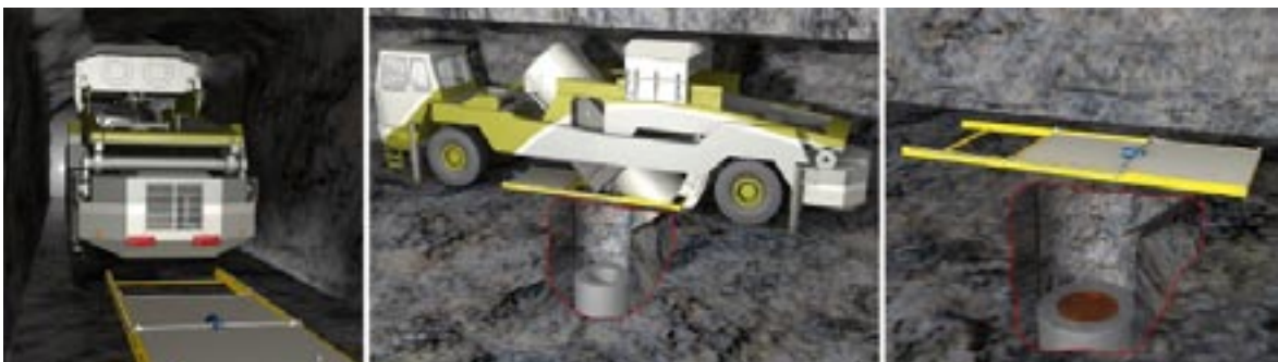
Figure 2-5. Deposition of canister. Left: Canister placement machine. Center: Insertion of canister. Right: Gamma-gate placed over the deposition hole.
