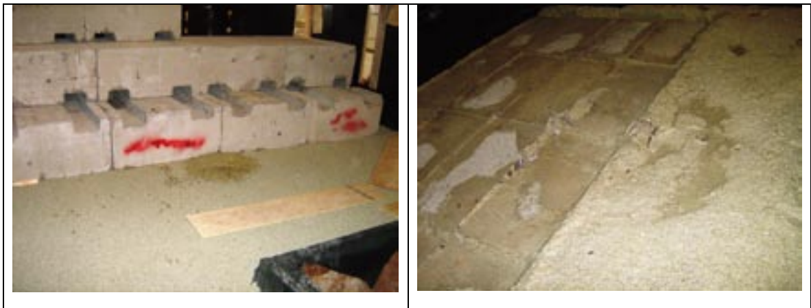
Figure 5-9 Left: Water from the injection point in the middle found a way up on the surface very soon. Right: The surface in front of the pile was strongly affected by the high water inflow (1 l/min). Also in this test dry areas could be found under the blocks.
