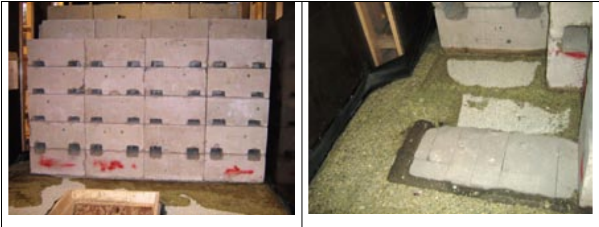
Figure 5-11 Left: During the installation of backfill blocks, water started to flow up on the surface from both sides of the tunnel. Right: After finishing the test it was observed that there were large dry parts under the blocks but the material under the joints was wetted. The bentonite blocks placed under the first row did not affect the stability.
