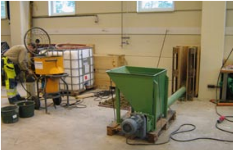
Figure 4-17. Pilot test using an auger for placing pellets.
