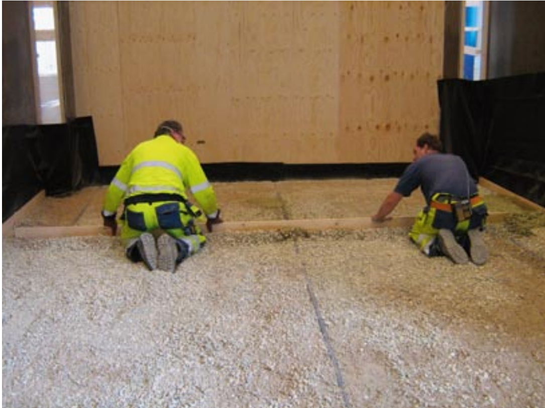
Figure 4-1. Preparation of the bottom bed using Minelco granulate.
