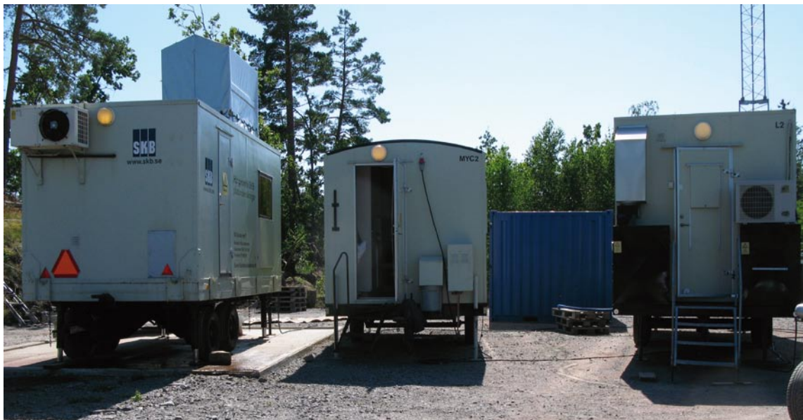
Figure 4-1. The mobile units used at KLX15A; from left hose unit with downhole equipment, a unit for computer work and laboratory unit.
