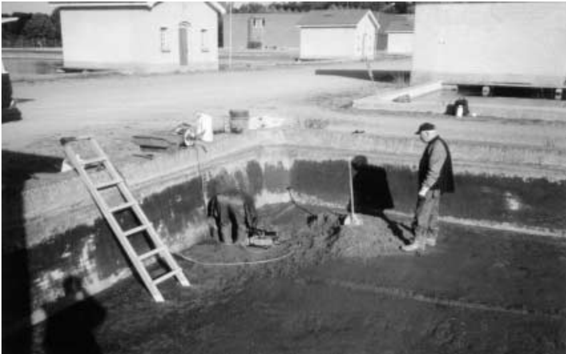
Figure 1. Basin at Norsborg when emptied for exchange of filter sand. One drill core was taken above and one from below sand layer.
