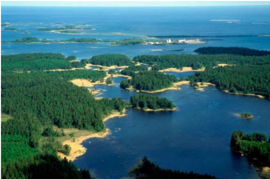
Figure 11-4. The central parts of the Forsmark candidate area, viewed from the south-west with Lake Bolundsfjärden in the foreground and the SFR buildings in the background.
