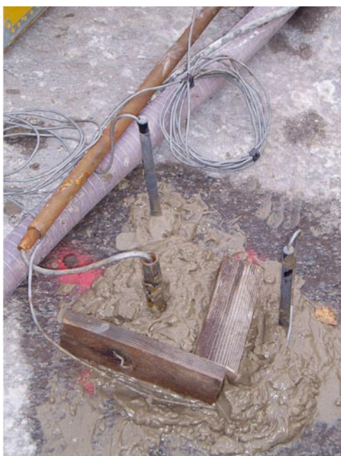
Figure 3-11. Multi-probe measurements in progress.
