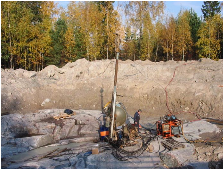
Figure 3-2. Drilling at location for large-scale experiment.
