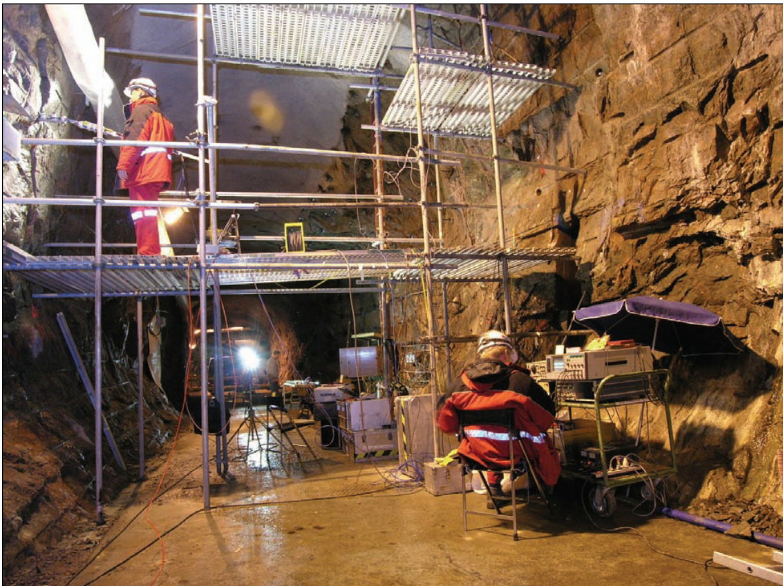
Figure 4–1. Ultrasonic measurements with the BGR mini sonic probe in the TASQ tunnel.
