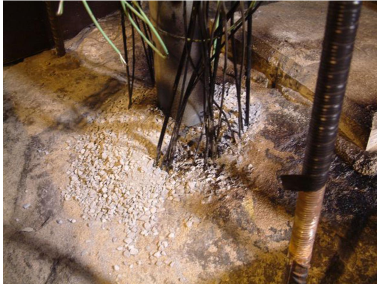
Figure 19. The uppermost 10 cm of the slot in all three packages were filled with granulate instead of sand. The granulate will quickly seal the package from water leaking into the hole from the tunnel. A small amount of granulate was also placed on top of the package
