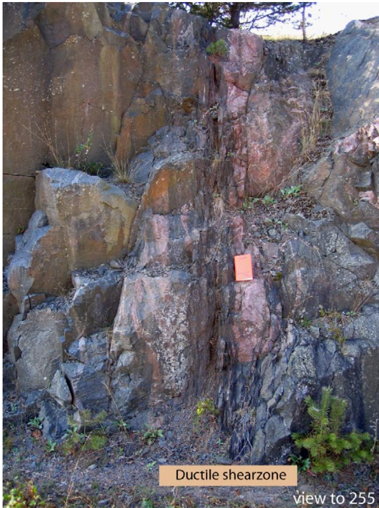
Figure 6-21. Steep protomylonitic shear zone in the outcrop opposite to the western entry of Block 3. Granitic slivers are visible in the deformed part.
