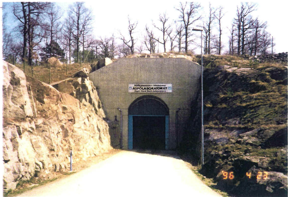
Figure 0-1 Tunnel entrance at Simpevarp.
