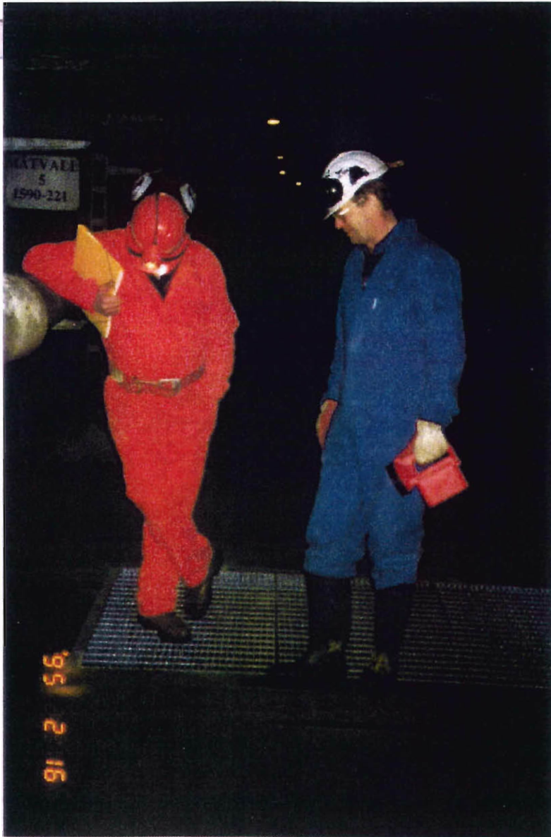
Figure 4-6 Grating on top of a sealing dam.
