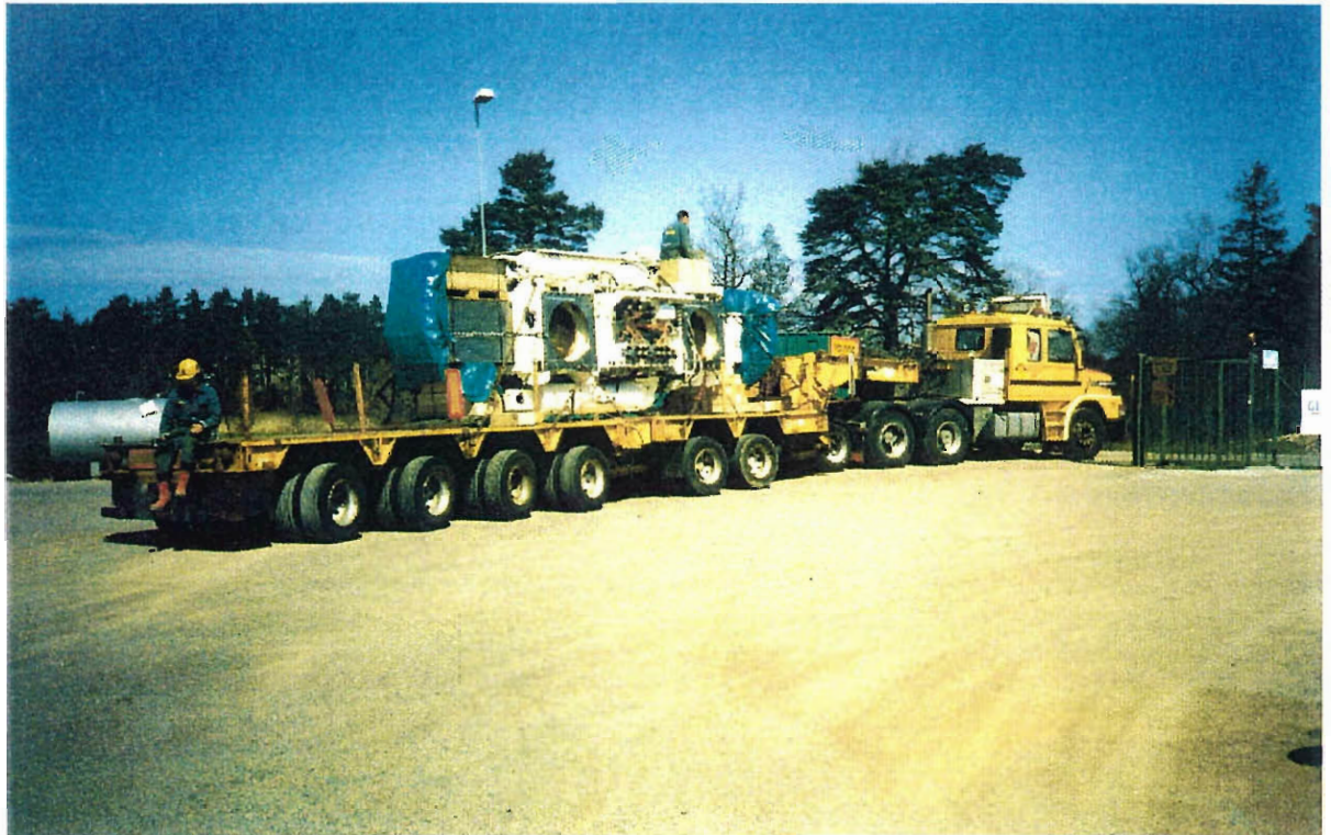
Figure 3-8 The 50 metric ton "main body" on a trailer at site.
