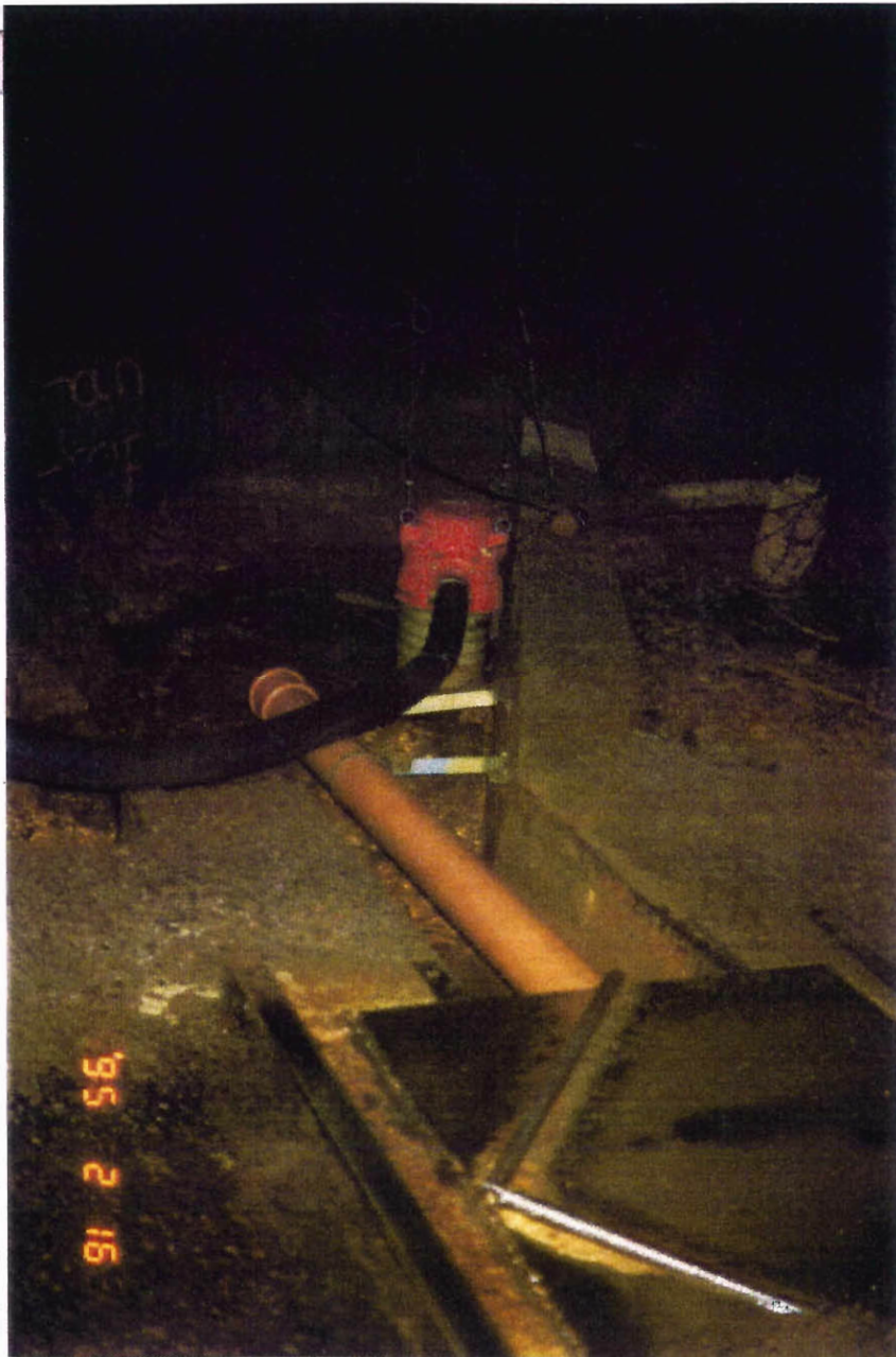
Figure 4-7 Collecting dam and pump at section 1/033.
