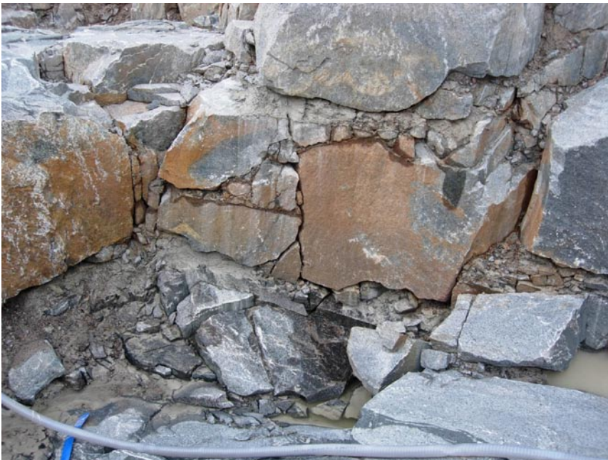
Figure B-2. Heavily fractured bedrock. Two subhorizontal sediment-filled fractures can be distinguished.
