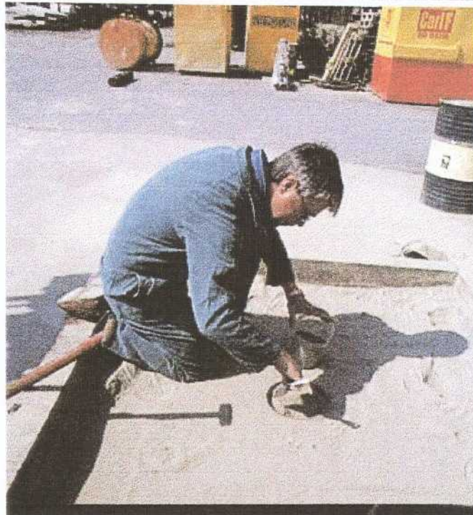
Figure 8 b. Field test arrangement. Upper: 400 kg vibrating plate. Lower: Volumeter for determination of density (Intergrund AB).
