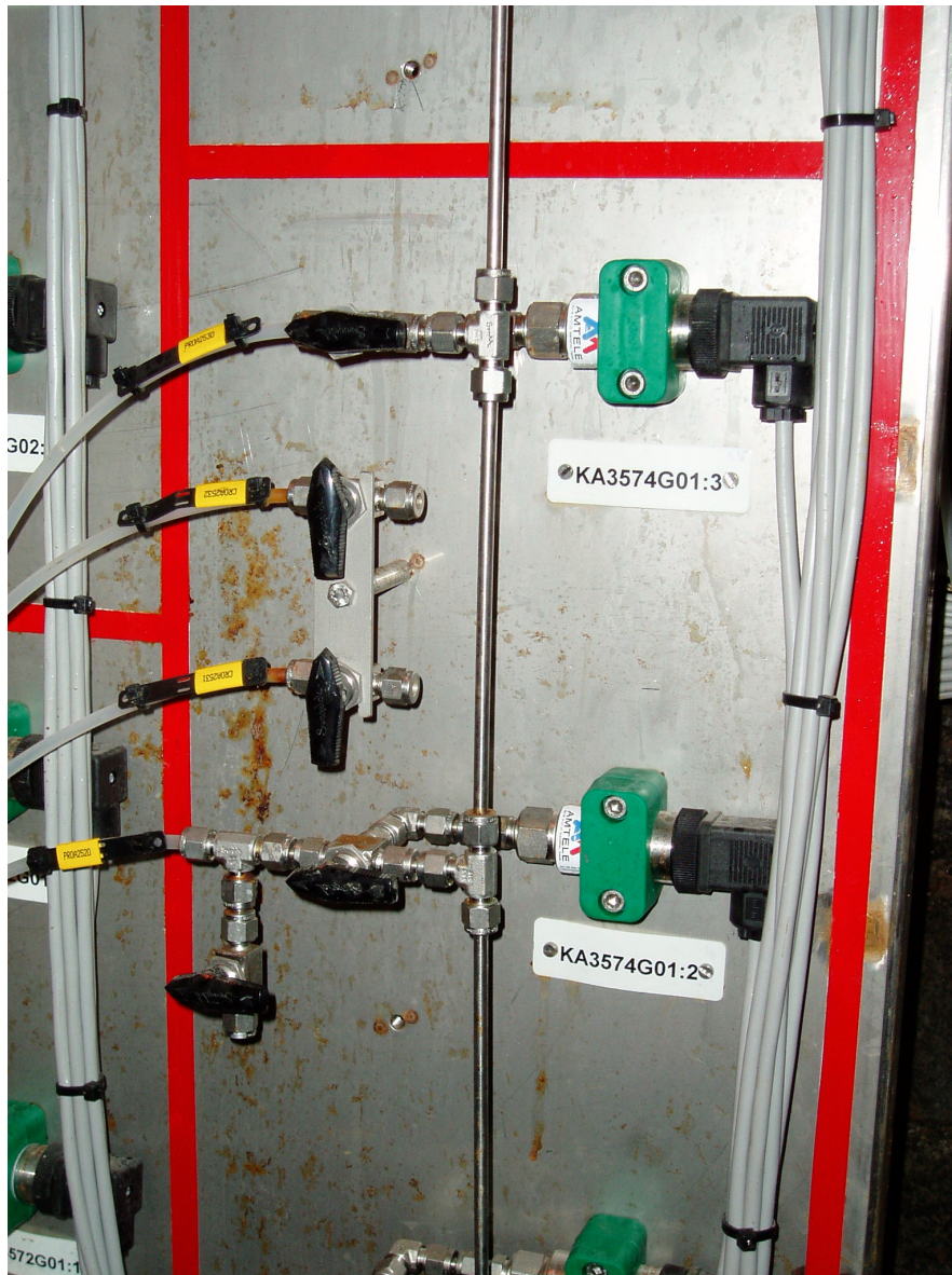
Figure 4-2. Pressure transducers connections.
