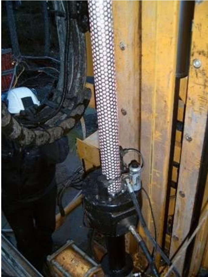
Figure 7-5. Jointing of two 2.5 m long units at Olkiluoto.
