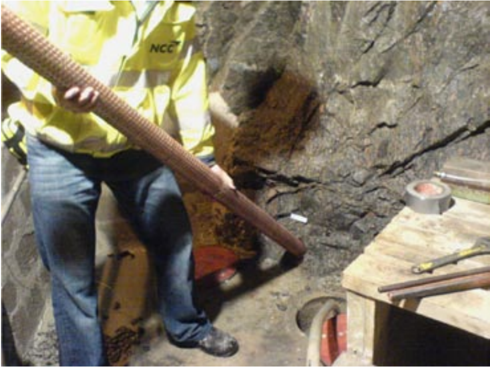
Figure 3-7. Placement of the plug of “Basic” type.
