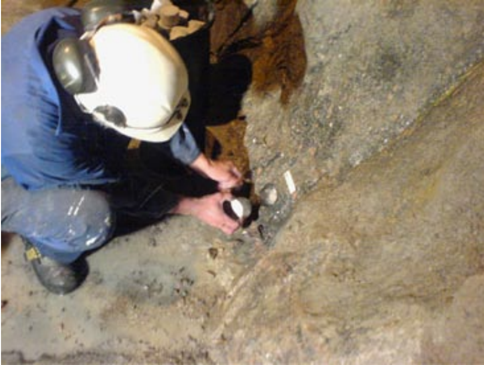
Figure 3-11. Manual placement of the clay components of the Container Plug. The hole into which the hand-held clay piece is being moved is just below the white label.
