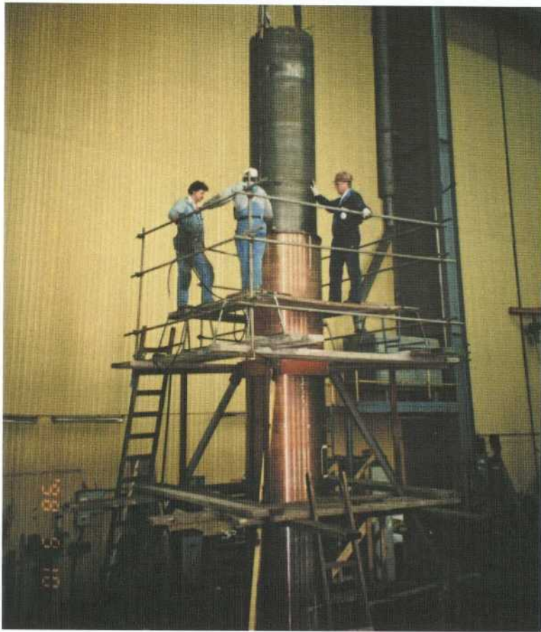
Figure 4-11. The assembling of a complete canister, C 3. The insert (I 10) is lowered into the copper casing, (T 9 and TB 3).
