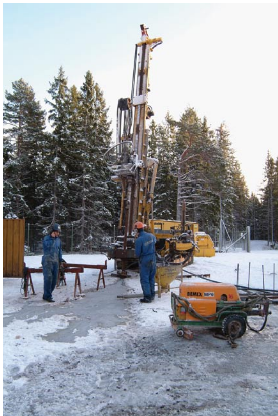
Figure 3-1. The Puntell percussion drilling machine in operation on borehole KFM02B.
