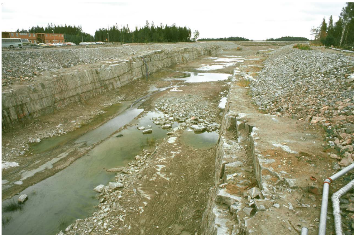
Figure 4-27. Picture from the construction of the 13 m deep and more than one kilometre long canal between the Baltic Sea and the nuclear power reactors. The horizontal fractures/ sheet joints are encountered along the entire excavation. There are several “beds” of extensive sheet joints on top of each other. The picture is taken from the southern side of the canal where the bridge crosses the canal between HFM20 and HFM22, see Figure 4-2. Reproduced from /Carlsson and Christiansson 2007/.
