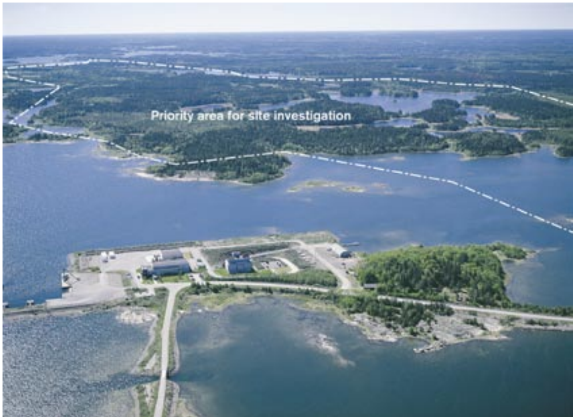
Figure 2-1. Overview of the Forsmark area seen from the Baltic Sea towards south.
