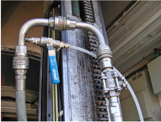
Photo 7. Top of test string with shunt valve and nylon line down to the pump basket.
