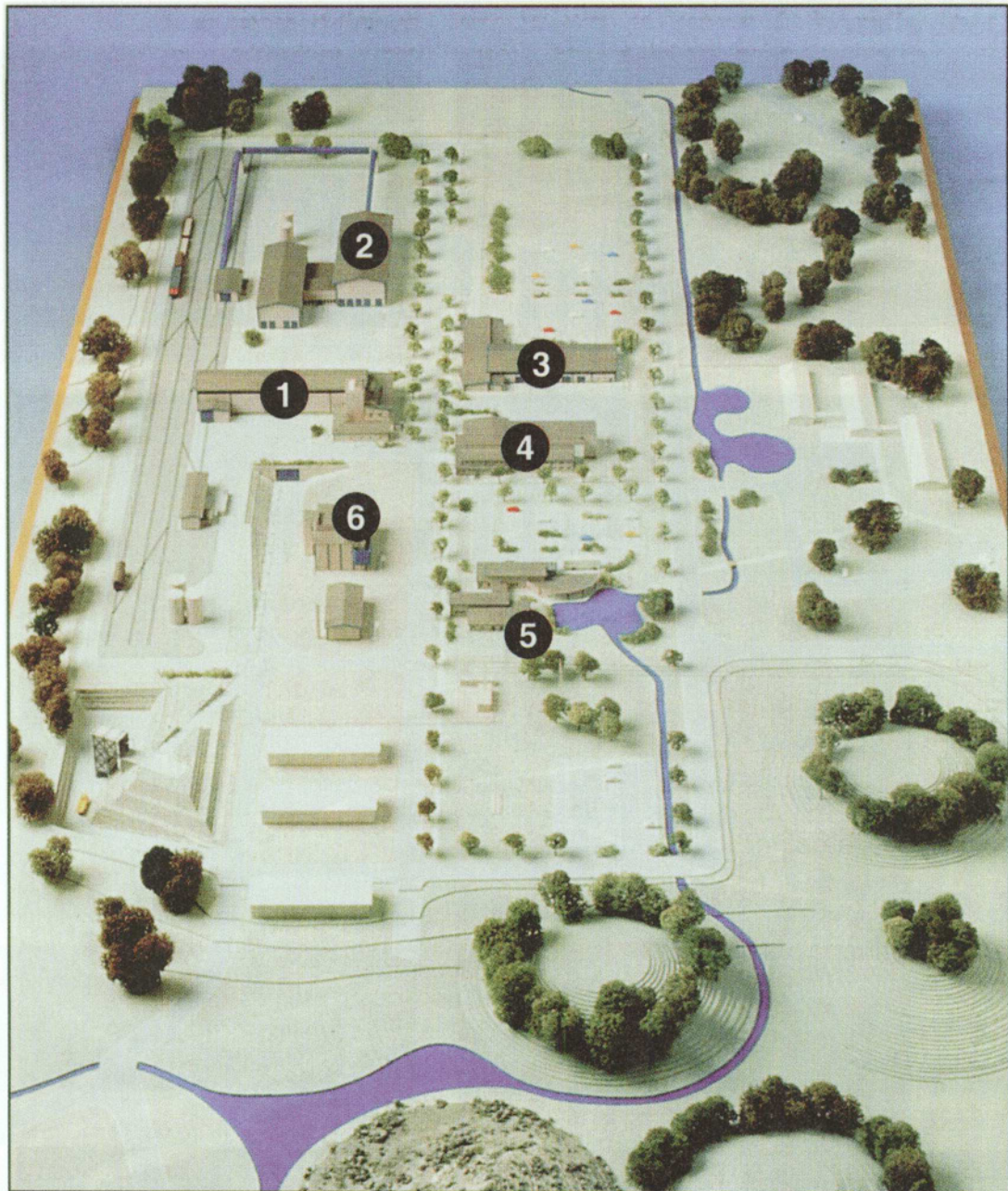
Figure 6-2. A possible layout of the deep repository's surface facilities. The example assumes flat ground and a railway connection to the facility.
